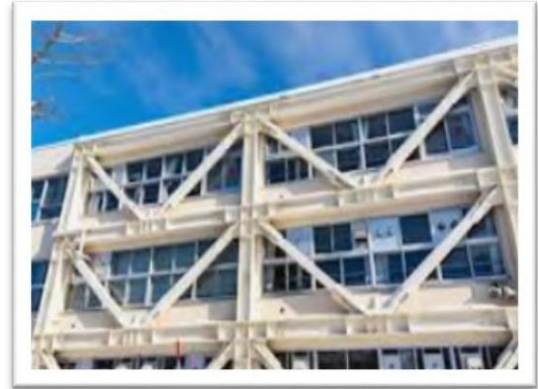
Figure 73: Seismic retrofitting
