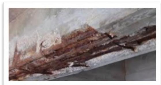
Figure 49: corrosion in slab
